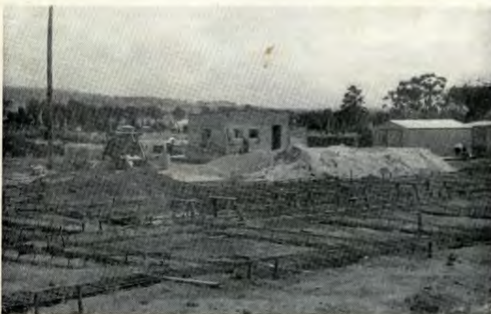
The New Men's Dormitory Under Construction
